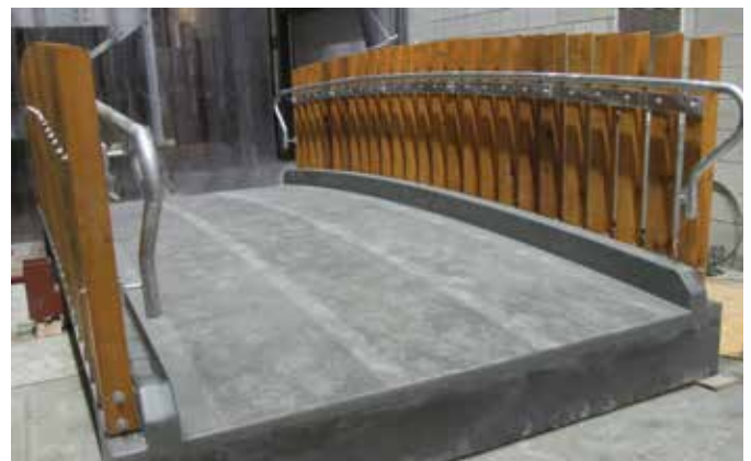
Fig. 4: As final preparation before shipping to the jobsite, wooden and steel railings were attached to the UHPGC curbs
